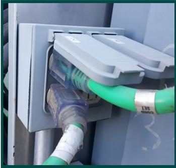
**ISSUE:** Sometimes our heat trace is unplugged from the outlet to make room for an engine block heater. Make sure all lines are plugged in.
