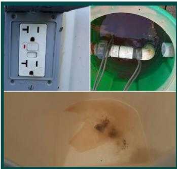
**ISSUE:** The toilet seems to be backing up and not flushing. This could be a sign that the GFCI has tripped or the lift station outside of the skid house is frozen.
