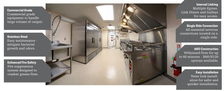
HB Rentals' A60 ABS/USCG Galley Module, certified to ABS and USCG regulations, is equipped with stainless steel commercial grade appliances to handle any volume of cooking. Unique safety features designed to combat grease fires are standard on the Galley.
